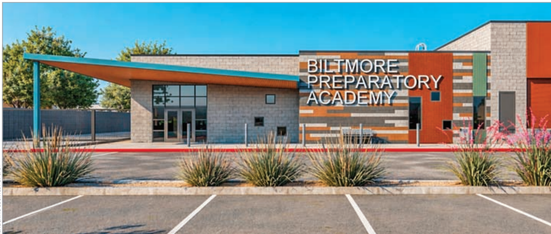
Four new buildings totaling 82,000 square feet of space are slated to be completed in the 2027-28 school year, but the school will be open during construction.
