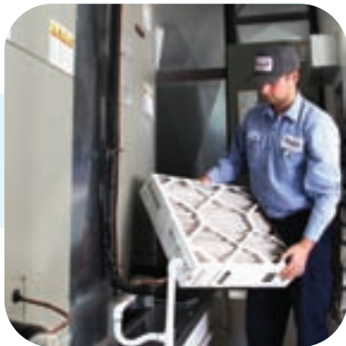
A/C – Heater Maintenance
