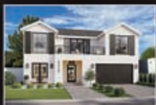
New Construction 4218 N. 45th Pl. $2,500,000
