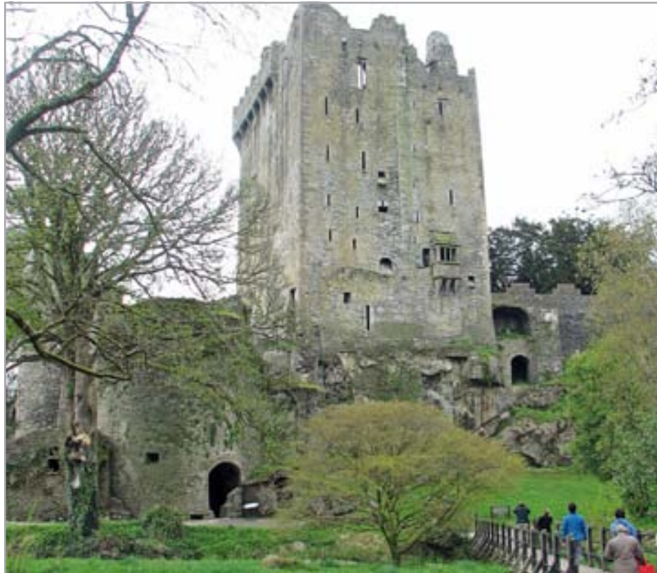
Blarney Castle has been torn down and reconstructed three times; this version was built around 1446.
