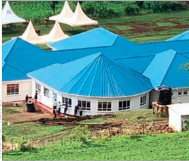
Love4Bukwo Regional Hospital under construction.
