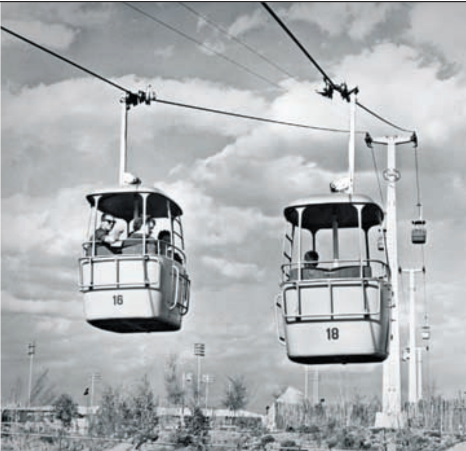
Spanning the width of the park, the 80-foot high Sky Ride could accommodate 900 passengers per hour in its 28 cars. The ride was built in Switzerland by Von Roll Manufacturing, for $290,000.
