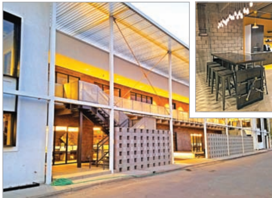
The Grid.Works has an open concept design featuring glass-walled offices and conference rooms.
