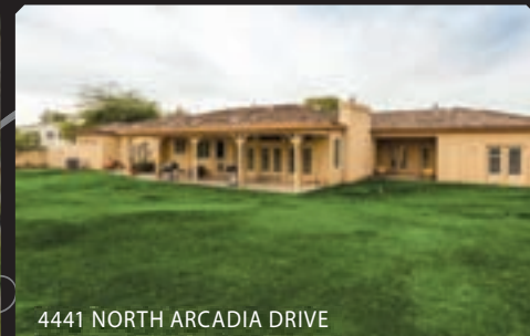
4441 NORTH ARCADIA DRIVE
