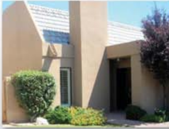
6305 E. 30th Court Phoenix 85016 - $2,200 mo. Awesome, private, total renovation of this 3bed/2bath home situated directly on the Arizona Biltmore Golf Course.
