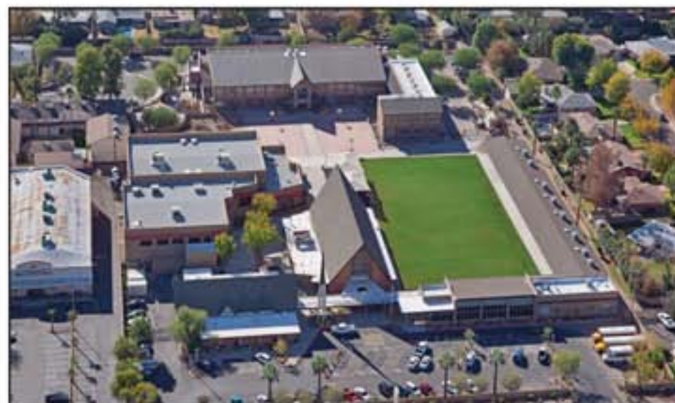
Christ Lutheran School has just finished construction on its fourth building – in 5 years.
